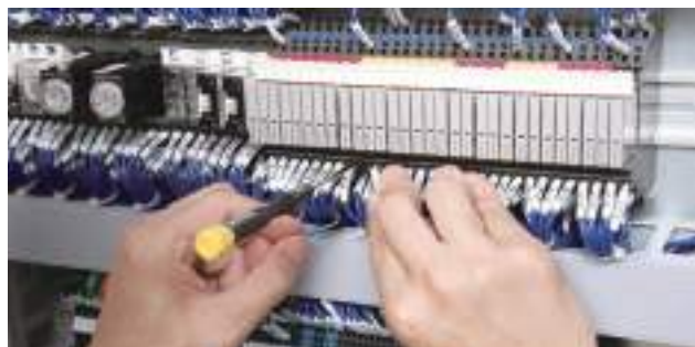
Reducing Wiring Work ..... P8
