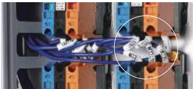
Previous Hard wiring in the narrow space by the interference of wires due to the screw terminals requiring wiring in vertical direction....
