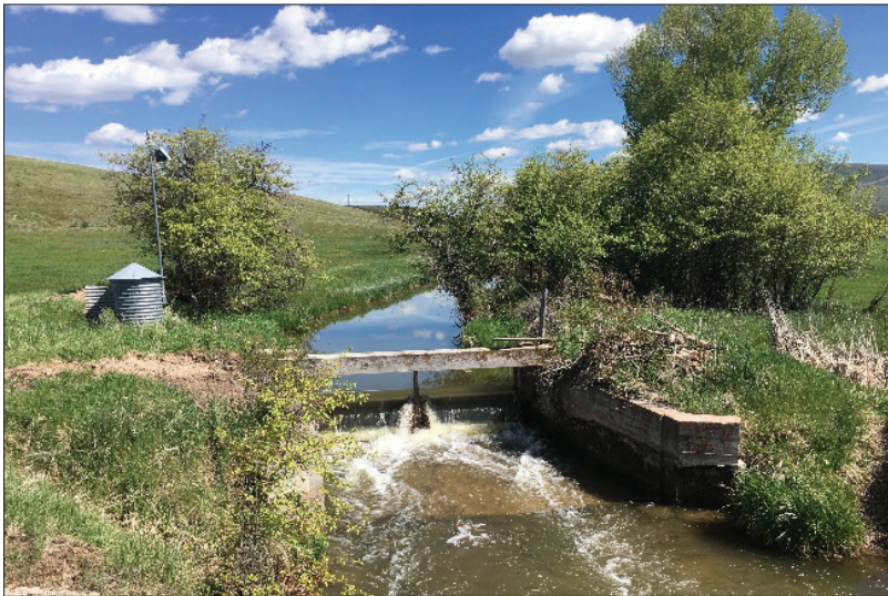
Site 2, corrugated stilling well next to a 12 ft wide weir
